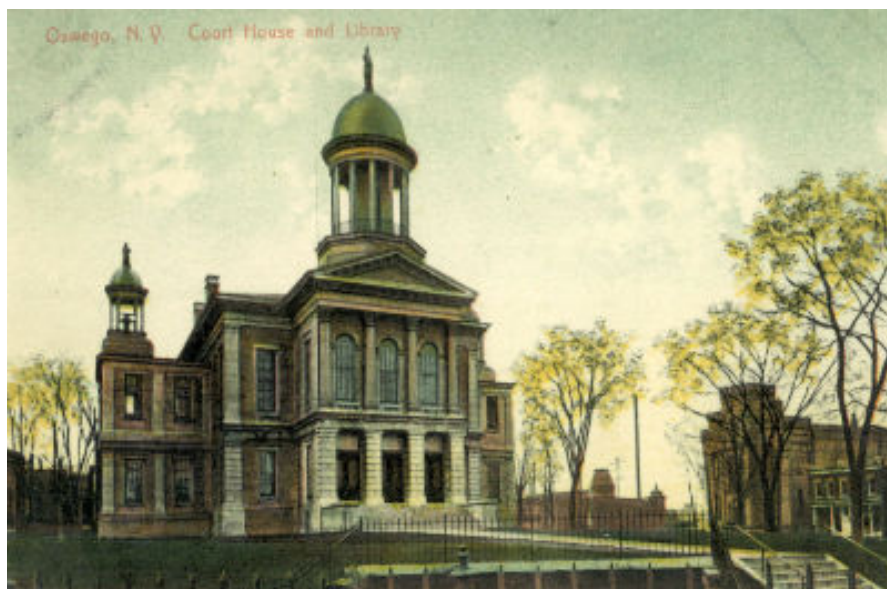
Photos of the Oswego Courthouse. 28
