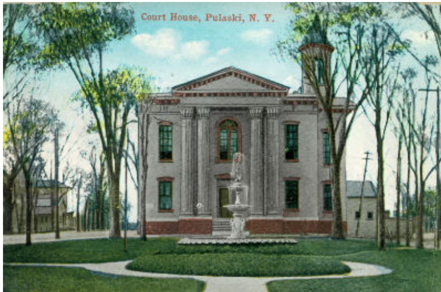
The Pulaski Courthouse. 18
