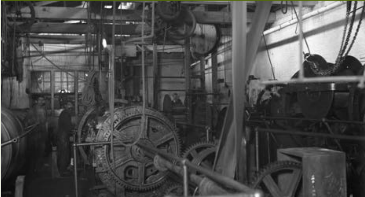
Wire rope machinery without protective guards fills a room at the Waterbury Wire Cable Manufacturing Co. in Brooklyn, NY c. 1912. New York State Archives. Factory Investigating Commission. Glass plate negatives and photographic prints of factory and housing conditions. 1911-1912. A3029-78, Box 5, Folder 7.
