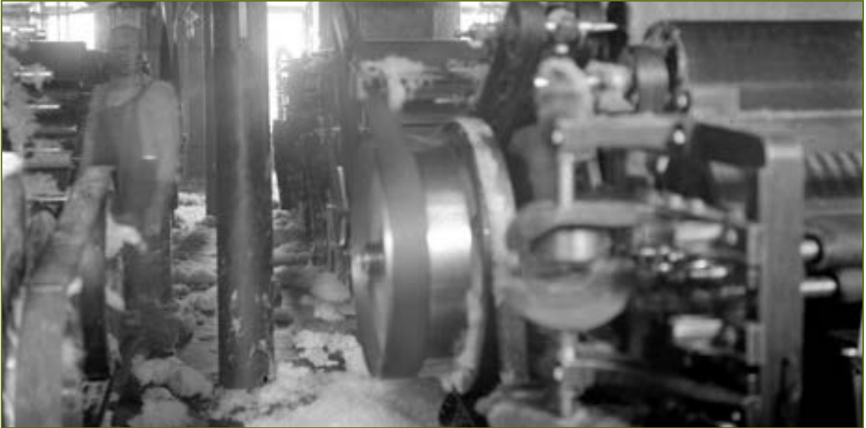
A worker stands beside machinery for carding cotton to manufacture men's underwear at a Union Mills plant in Hudson, NY, 1912. Cotton floss covers the floor and machinery; an investigation found that exhaust fans would remove the floss and reduce the risk of fire. New York State Archives. Factory Investigating Commission. Glass plate negatives and photographic prints of factory and housing conditions. 1911-1912. A3029-78, Box 4, Folder 11.
