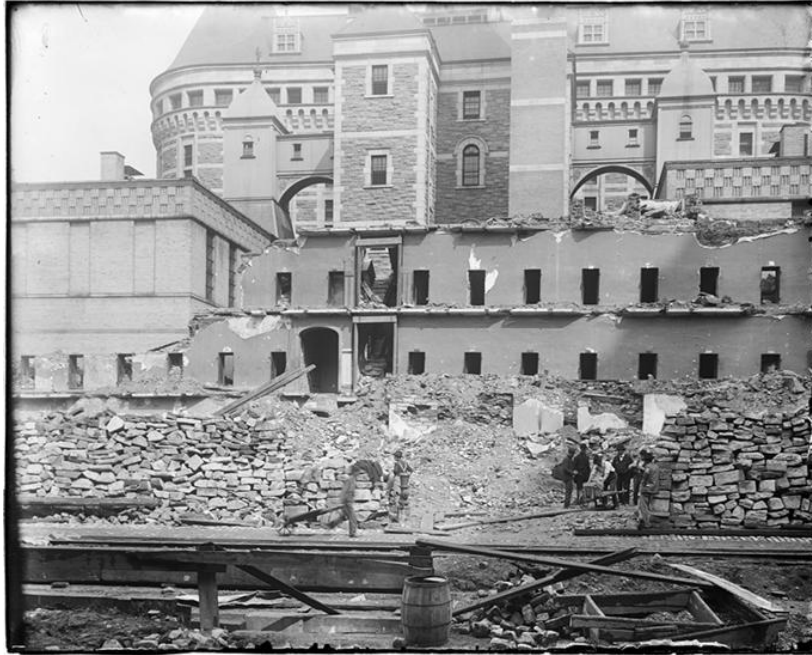
Demolition of the original Tombs Prison, circa 1902. The successor Tombs can be seen in the rear. Robert L. Bracklow / Museum of the City of New York, 93.91.338.
