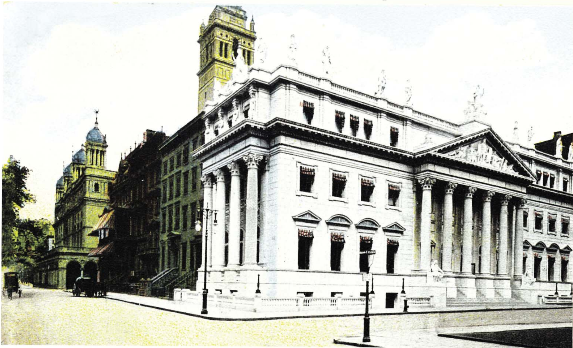
THE OPENING OF THE NEW COURTHOUSE: The Court took possession of its new home at 27 Madison Avenue on January 2, 1900
