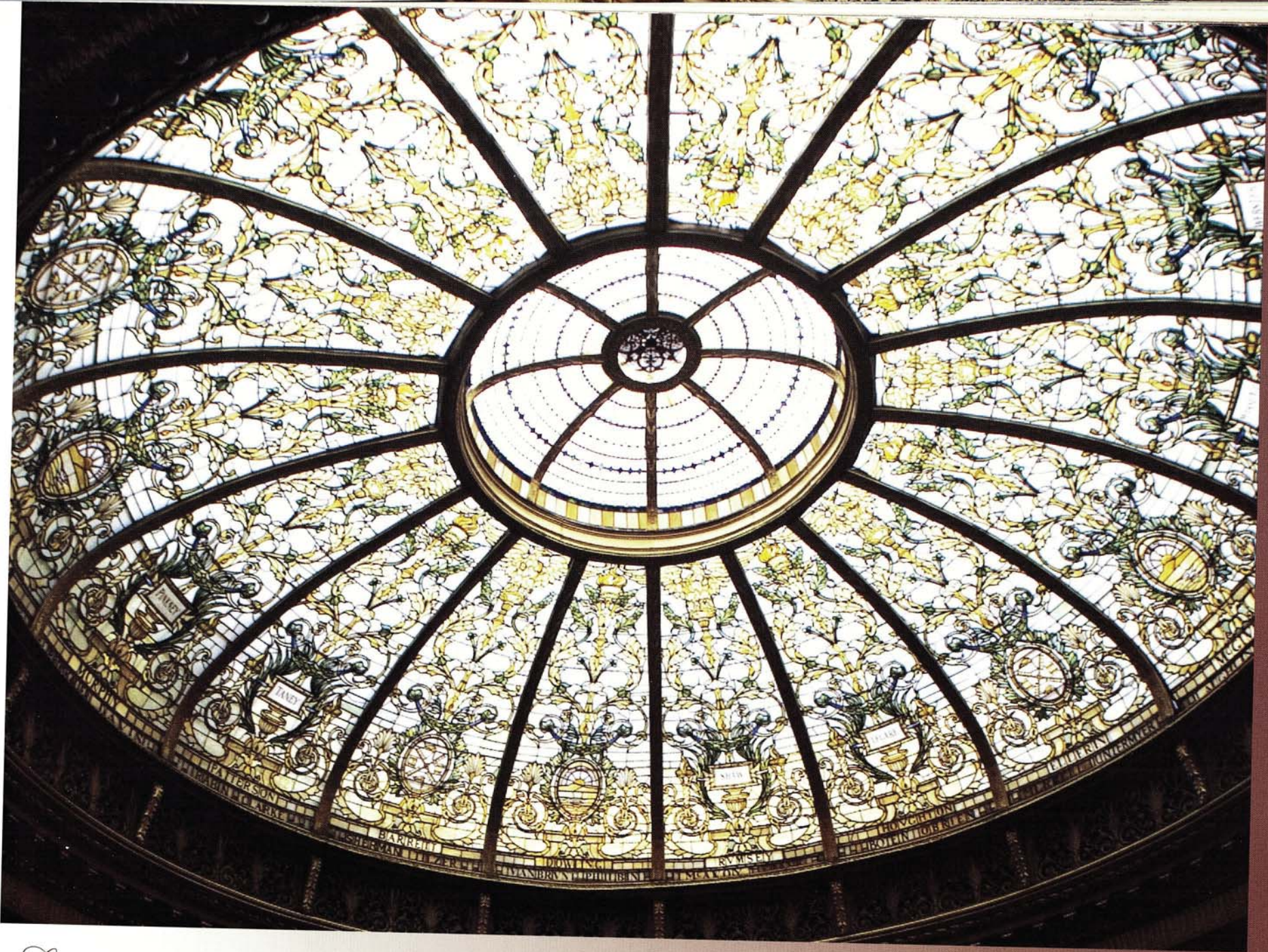
S TAINED GLASS DOME: A spectacular stained glass dome is set in the ceiling of the Courtroom. The dome is composed of 16 radiating stained glass panels, with ornate floral and fruit designs.
